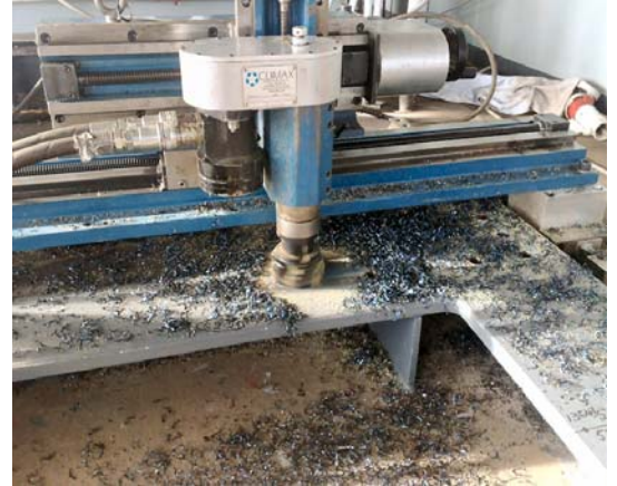
On Site Milling Of A Support Base To A Known Datum
