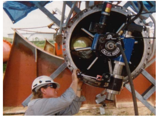
Setting Up The Flange Facer to Machine A 650mm Ø Flange
