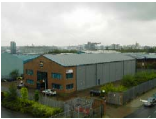
The New Factory
