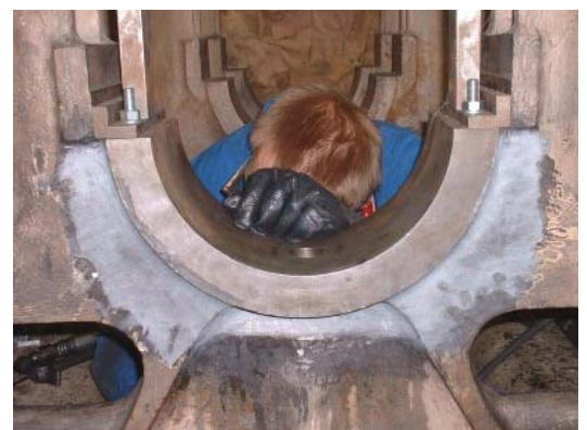
Finished Repair After Hand Dressing
